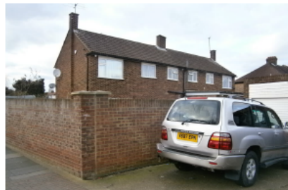
REAR WINDOWS ADJACENT TO THE SITE
