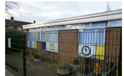
EXISTING BUILDING ON THE SITE
